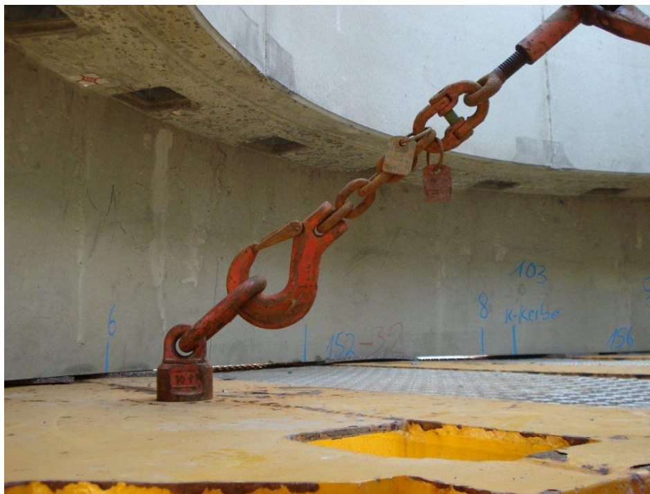
Figure 7: Example for fixation tooling for the connection-element during the transport
