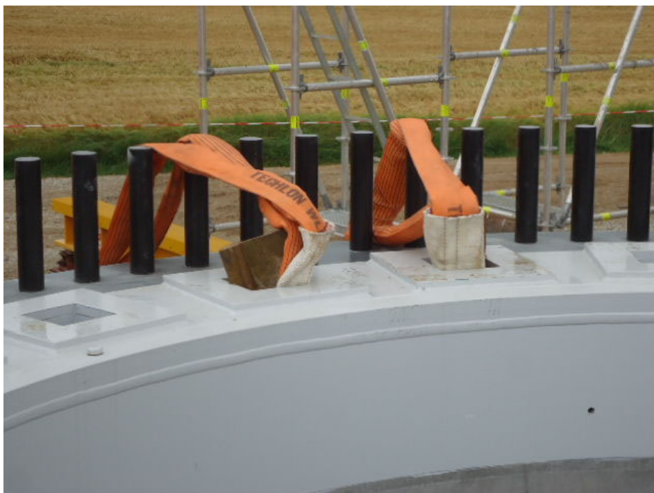
Figure 9: Upper edge of the adapter with implemented slippage
