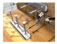
Fixing of the anchor channel to timber formwork with nails through the prefabricated holes in the back of the anchor channel
