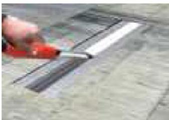
Removing the foam filler with a hammer or a hook
