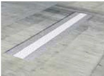
During casting the concrete has to be compacted properly around the channel and the anchors
