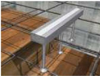
Fixing of the anchor channel from above directly to the reinforcement, attach the channel by wire binding
