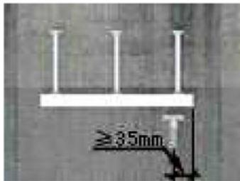
Positioning of the special screw: at the channel ends a minimum clearance must be maintained ( $\geq 35\text{mm}$ )
