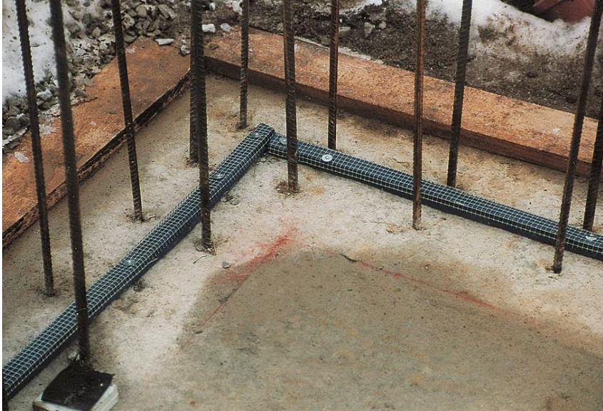
Example for installation with grid and nails
