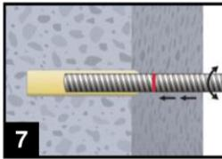
7. Push the reinforcing bar into the anchor hole while turning slightly to ensure positive distribution of the adhesive until the embedment depth is reached.
