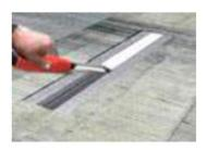
Removing the foam filler with a hammer or a hook
