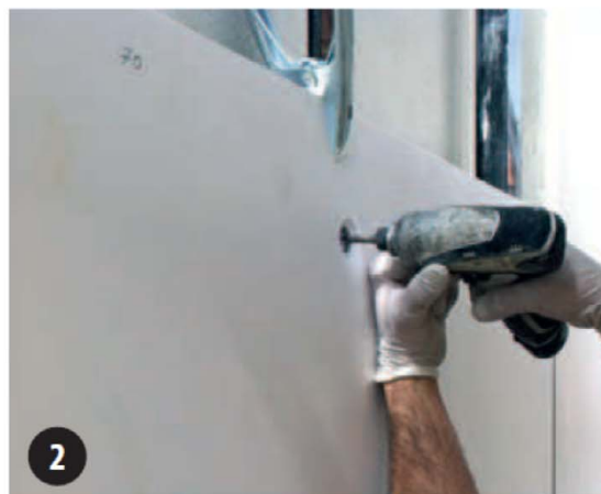
2 Insert the K-Fix cap in the bore hole and screw in the K-Fix cap and the substructure with the K-Fix screw.
