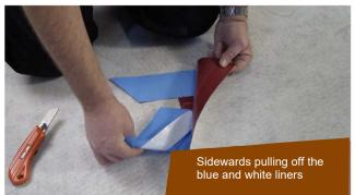
Bonding of the lateral/cut seams using the double-sided adhesive tape TP10 and the swelling paste KD5 active:
