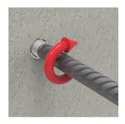
Approach the rebar to the coupler and start rotating.
