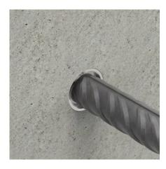
When the installation is completed: no threaded portion of the  $2^{nd}$  phase rebar is visible outside the coupler.
