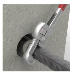
Use a standard wrench to tighten the rebar. For rebar with  $\varnothing \ge 25$  mm, use a minimum lever length of 0,80 m
