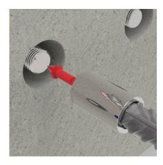
Check that the coupler is fully engaged on the 2nd Phase rebar.
