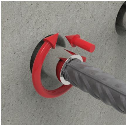
Approach the 2nd Phase Rebar to the 1st Phase Rebar until they are in contact, then start rotating the coupler.
